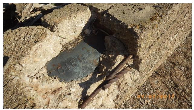
Figure 33. View of broken concrete exposing pipe and two kinds of rebar. Damascus Twist Rebar is present in the structure.
