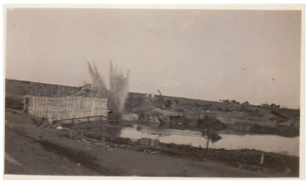
Figure 21. Blowing up southern abutment of the bridge. Date unknown. Courtesy of Stephen Vinson.
