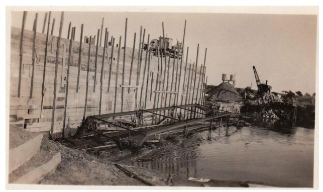
Figure 22. View of the bridge laying in the river channel. Date unknown. Courtesy of Stephen Vinson.
